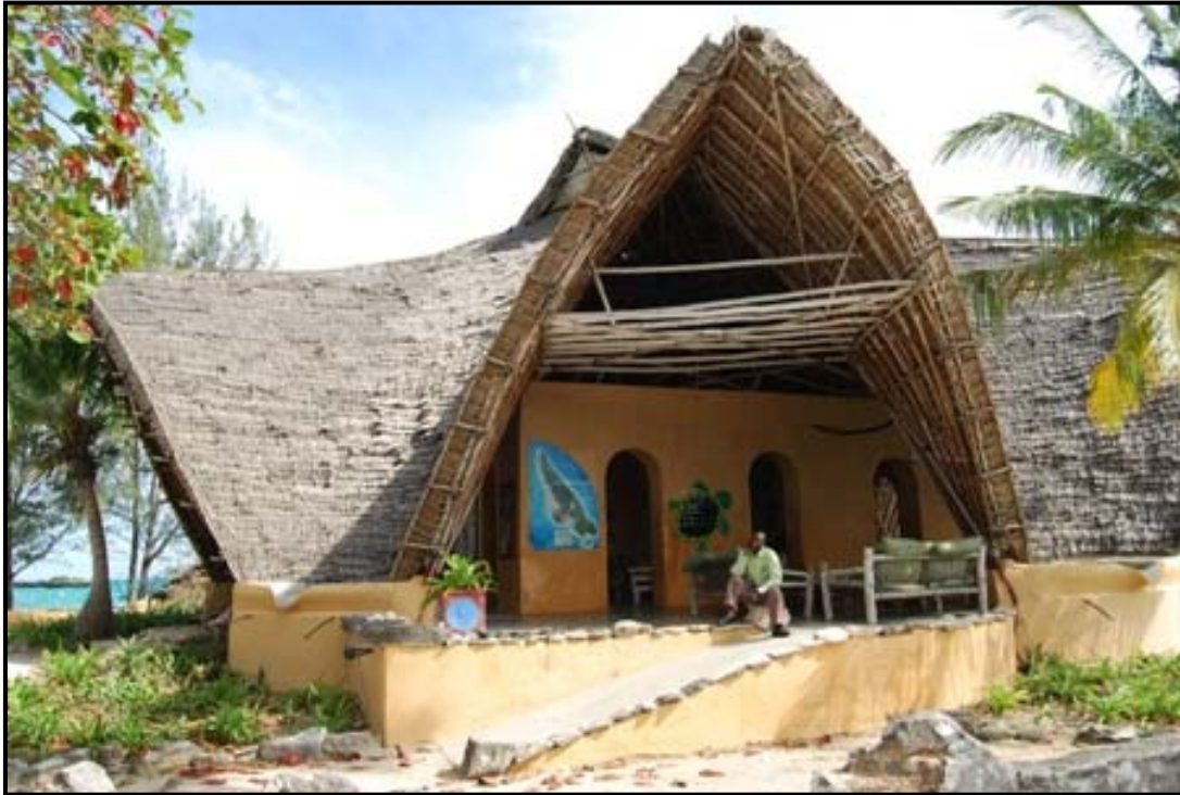
Chumbe Island Main Building
