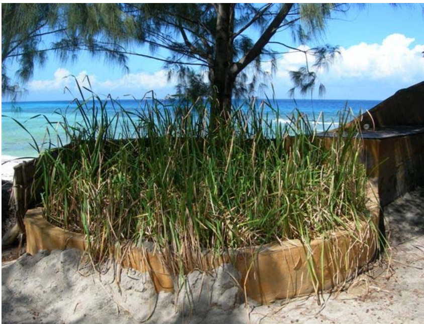
Picture 1. The new well-functioning grey water filtration system
